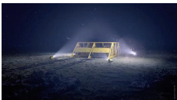
Åsgard subsea compressor station on the seabed - © Statoil ASA
