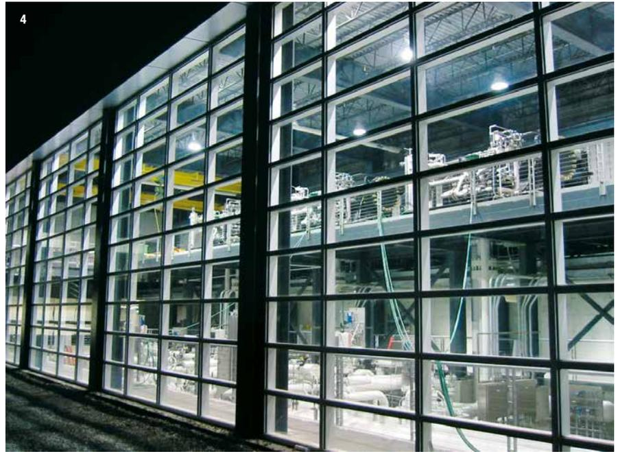
**4** The first three HOFIM™ units operating in a gas storage facility in New York State. The plant layout allows the three units to operate in parallel, but also two units in parallel, feeding the third unit in series for high-pressure ratio requirements. Each motor is rated at approximately 7 MW. Gas can be compressed from 55.2 bar up to a maximum of 220.6 bar.
